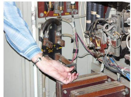
3. Turn on/clockwise both ENGINE SHUTDOWN switches
